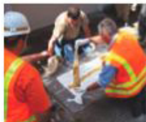
Prepare resin and patch
