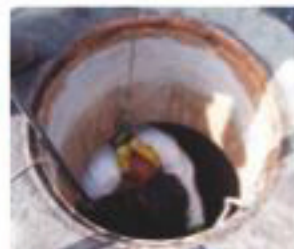
Push packer into sewer line
